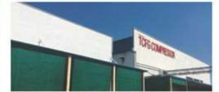
TCFG Compressor (Thailand) Co., Ltd. (Thailand)
