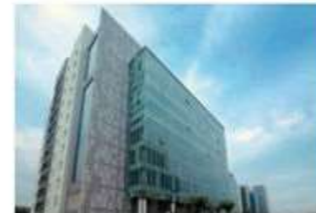
ABS Aircon Engineers Private Ltd. (India)
