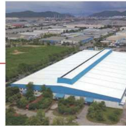
Fujitsu General (Thailand) Co., Ltd. (Thailand) Factory-2
