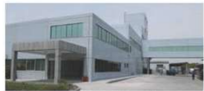
R&D center in Fujitsu General (Shanghai)
